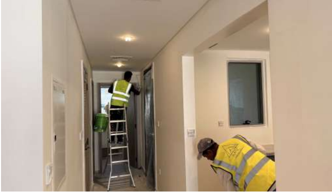
DAMAC LAGOONS / DUBAI — RECTIFICATION WORKS
