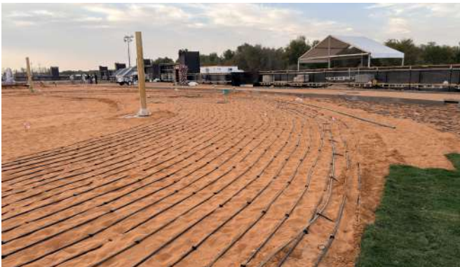
AL AIN / UAE — SITE INFRASTRUCTURE WORKS
