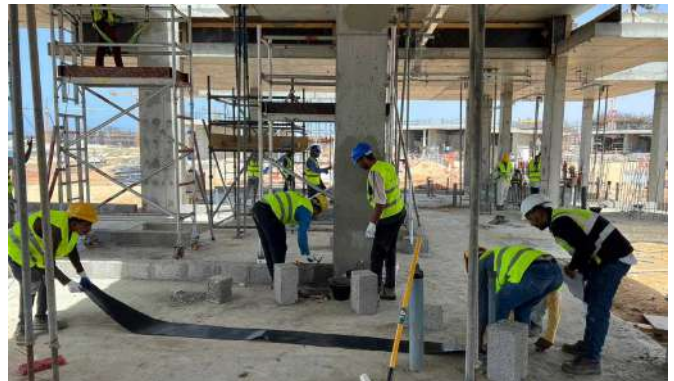
FOUR SEASONS — AMAALA / KSA — MASONRY WORKS
