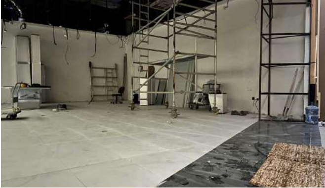
DERAAH / UAE — INTERIOR FIT-OUT WORKS
