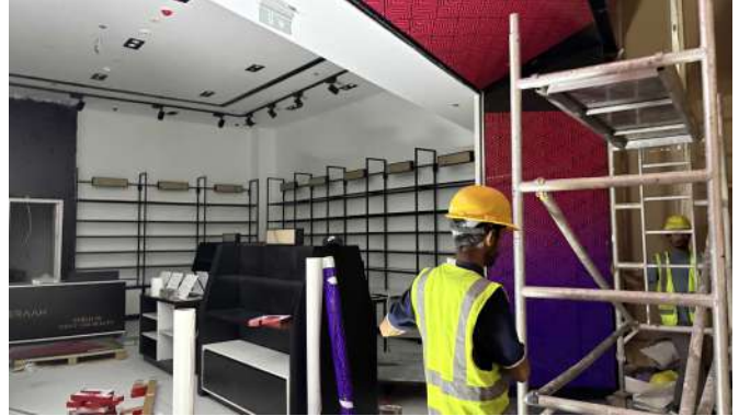
DERAAH / UAE — RETAIL FIT-OUT EXECUTION
