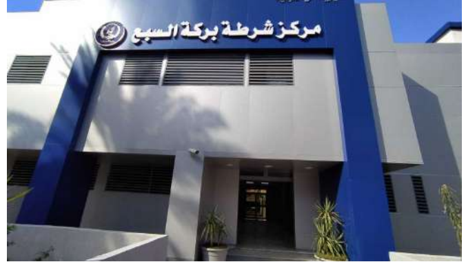
BERKET EL-SABAA POLICE STATION / MENOUFIA — MAIN FACADE
