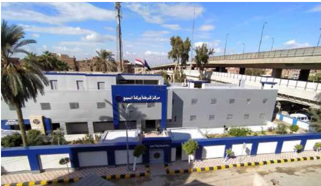
BERKET EL-SABAA POLICE STATION / MENOUFIA — GENERAL VIEW
