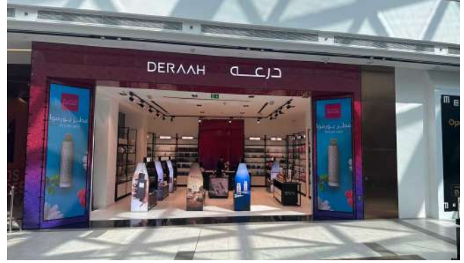
DERAAH / UAE — COMPLETED STOREFRONT
