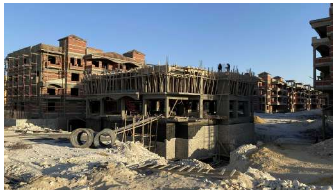
EGYPT / RESIDENTIAL CONSTRUCTION — STRUCTURAL WORKS
